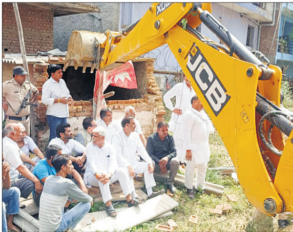
Sikanderpur villagers stall demolition work on Thursday. TRIBUNE PHOTO
